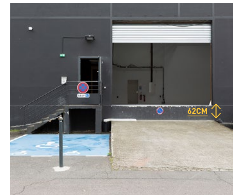
EXTERIOR ACCESS, 62CM HIGH STEP
